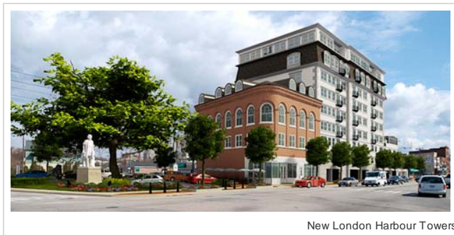
New London Harbour Towers
